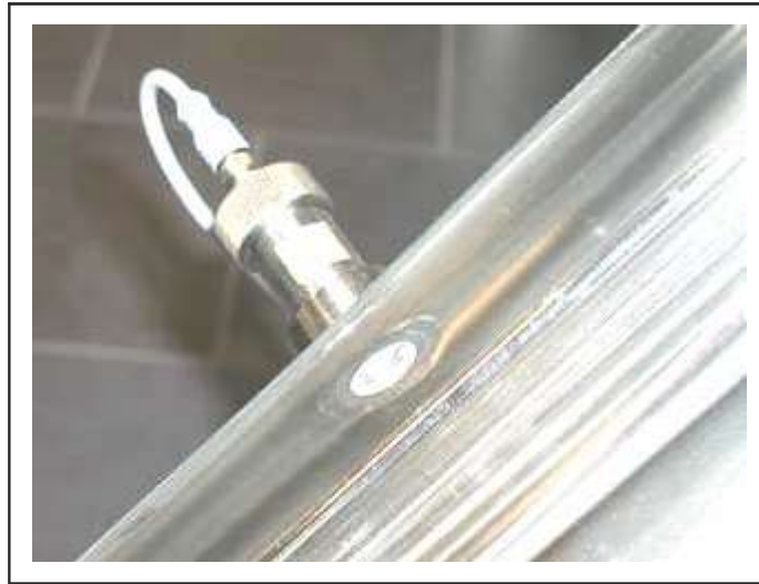
Figure 2.20. Example of a Dry UV Sensor Mounted on a UV Reactor
