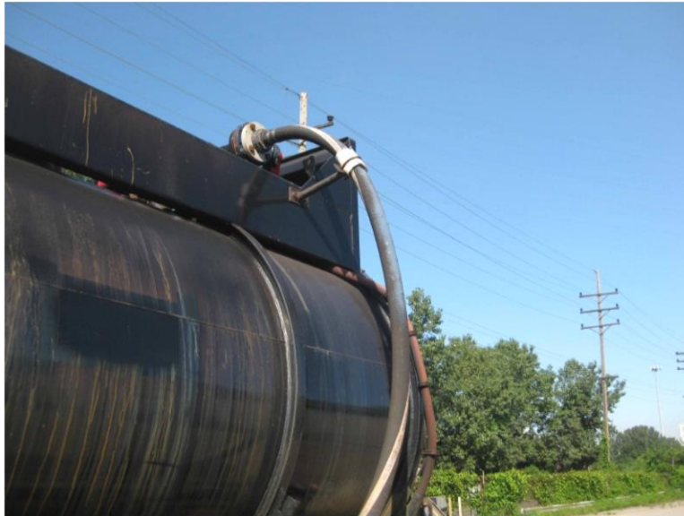
Figure 10- Miscellaneous in-line plumbing not protected
