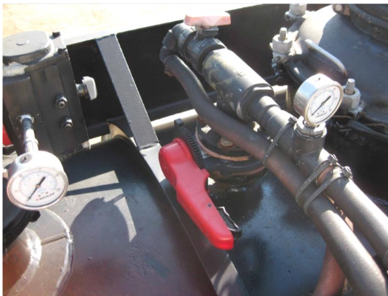
Figure 11- Miscellaneous in-line plumbing not protected
